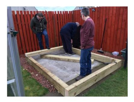
The sleepers are solid and really heavy, so they didn't need fixing to the floor, but once we got the basics of the frame cut and in positions, we did use huge carriage bolts to hold everything together.
